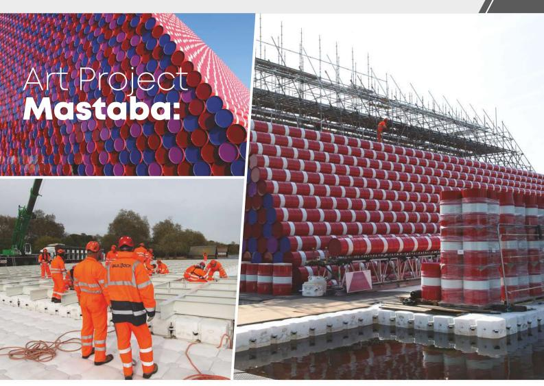
Deep Dive Systems under the brand of Buldock is taking part in constructing and anchoring of the floating structure. The Mastaba itself is a stack of 55-gallon barrels, numbering 7,506 in all, floating on the lake.
